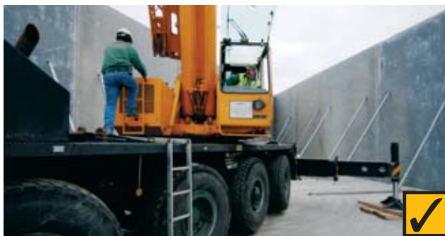
4.0 Person using a ladder working near the edge of a small structure – this situation is okay where the task is light and of short duration and the person can face the ladder and not over-reach.
