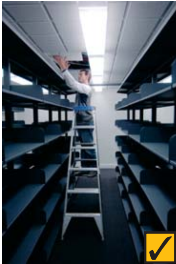
5.0 Ladder being used to inspect a ceiling space.
