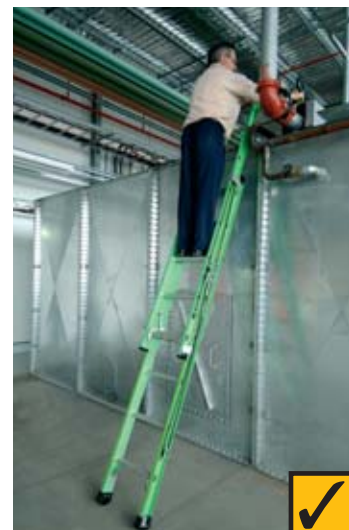
4.0 Person using a ladder working near the edge of a small structure – this situation is okay where the task is light and of short duration and the person can face the ladder and not over-reach.
