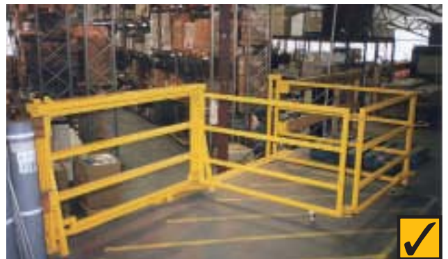
3.0 Mezzanine has a relocatable fence and sliding gate to ensure that no one is exposed to an unguarded edge at any time.
