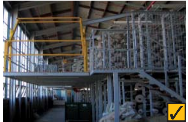
2.0 Access to a mezzanine via a stairway.
