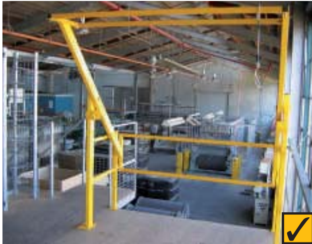
4.0 A safety gate that allows forklift access while separating personnel from the mezzanine edge. This design was a finalist in the Victorian WorkSafe Awards in 2003.
