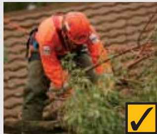
5.0 This VICSES worker is using a safety harness system.
