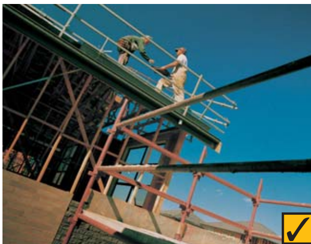
1.0 Adequate guard railing to roof work.
