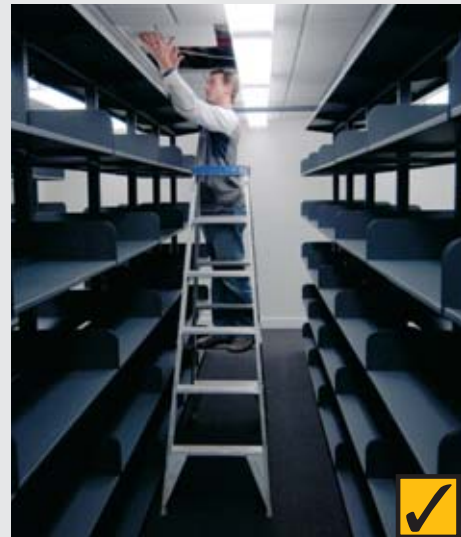
6.0 Ladder being used to inspect a ceiling space.
