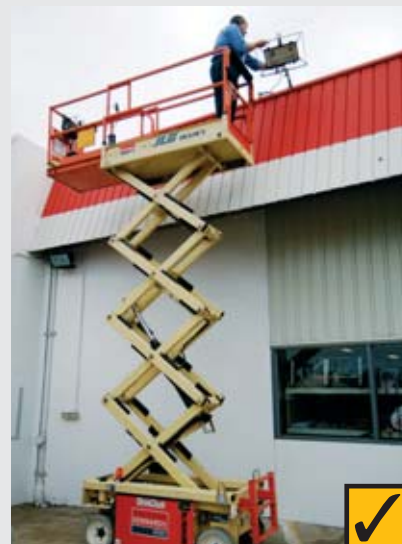
3.0 Undertaking work from an elevating work platform.
