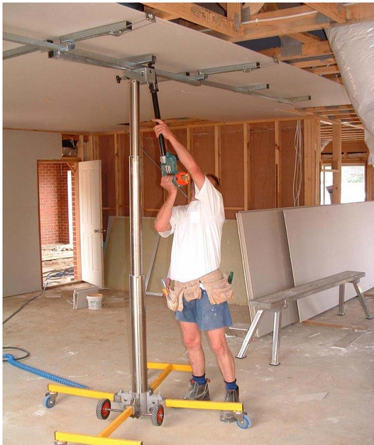
Pictured: a pneumatically-powered plaster sheet lifter with large extension screw gun
